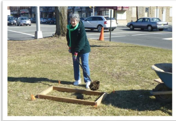
Rosemarie breaking ground for the sculpture foundation – April 1, 2014
